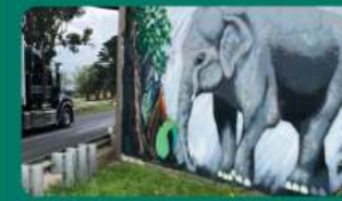
Stratford Rail Bridge Princes Hwy
