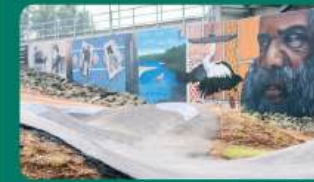
Rail Project Works Apex Park
